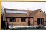
Domestic hot water and central heating (under) and swimming pool heating (summer) United Kingdom, 120 Tubes
